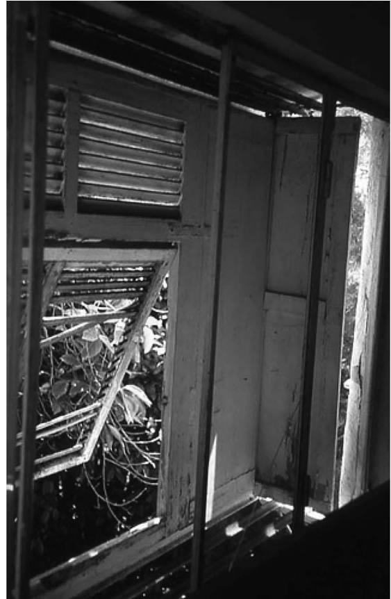
Figure 8 | Sliding shutters – as found by the author in 1998 Source: Ryan (1998)
